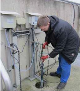
Employees of the wastewater treatment plant during the removal of the spectral sensor
